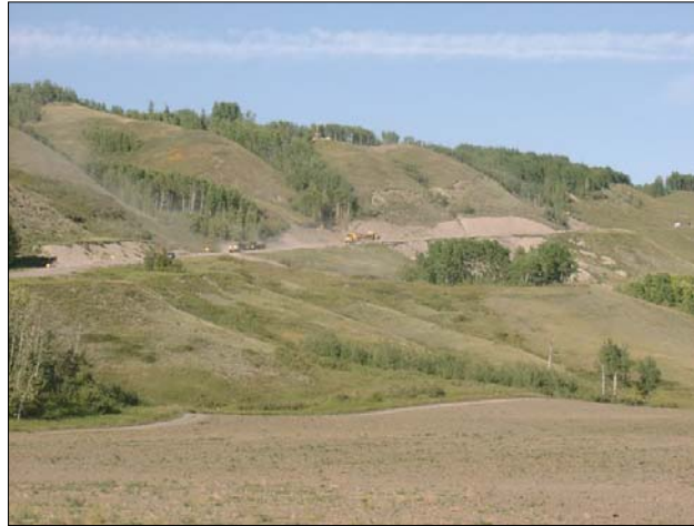
Road re-construction on Hwy 29 near Bear Flats
